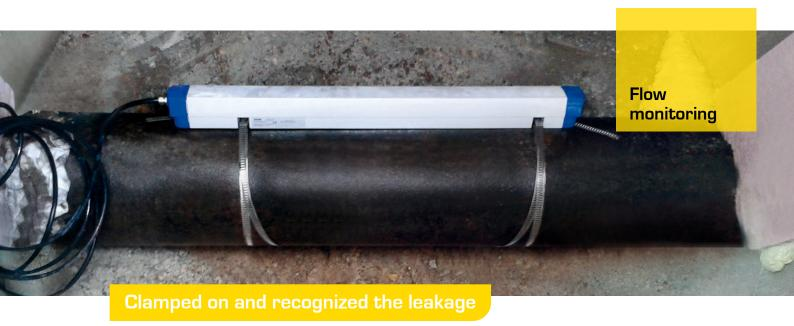
A lingering loss of water in the piping system is the fear of every water system caretaker. SPANGLER Automation has now enhanced a flow measurement system which can be installed on the outside of a pipe and sends data to a SCADA system.
